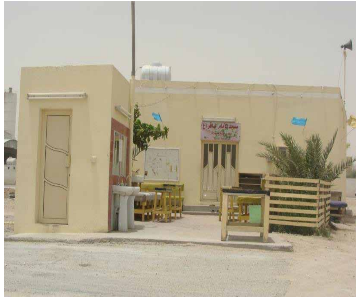
Al Imam Al Baqer Mosque in Nuwaidrat (Before Reconstruction)
