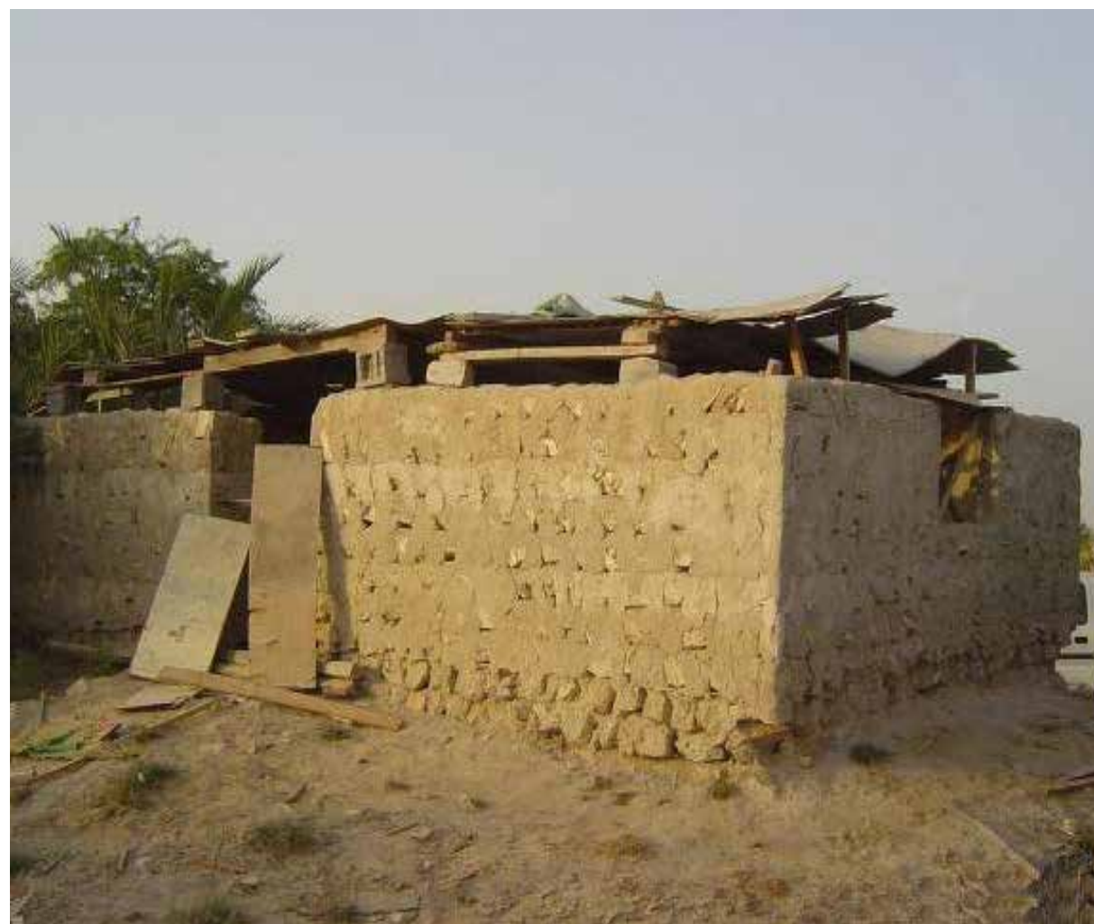
Imam Al Jawad Grand Mosque in Nuwaidrat (Before Reconstruction)
